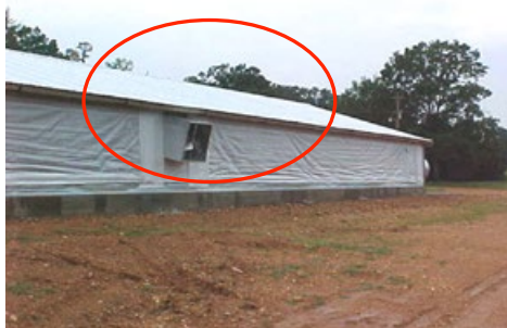
Minimum Ventilation Fan With House Closed
